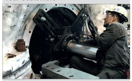
▲ Pipe cutters and weld preparation.
