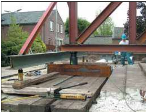
▼ P392 in action with RC256 cylinders.
