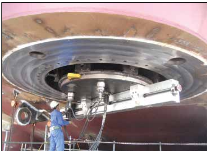
▼ Milling a ship thruster flange.
