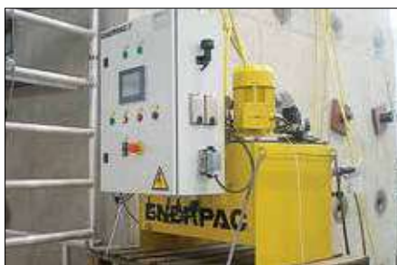
◀ Custom pumps with control packages.
