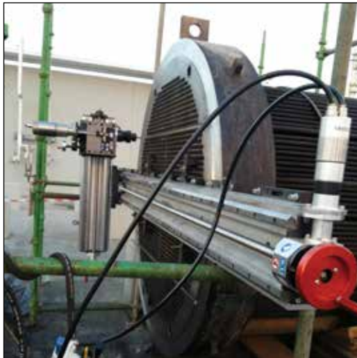
▼ MRY Milling machine on a heat exchanger.
