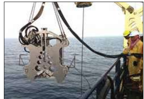
▲ MDWS Diamond Wire Saw lowered into sea.
