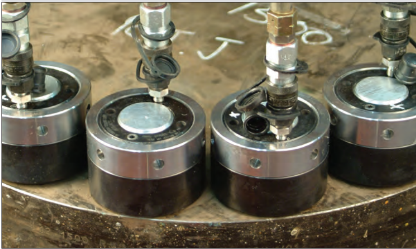
▲ Tensioning with hydraulic nuts.
