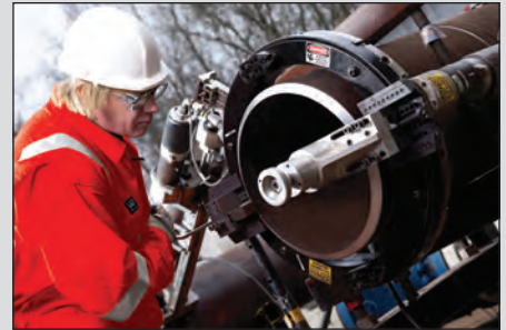
▲ Pipe cutters and weld preparation.
