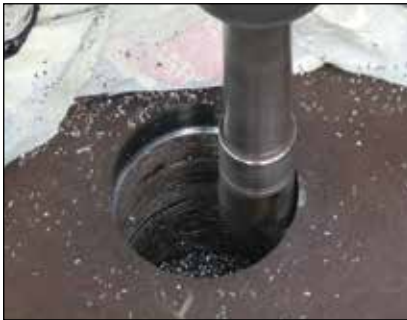
▲ Enlarging a hole
