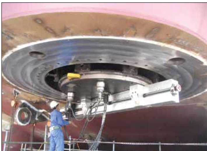
▼ Milling a ship thruster flange.
