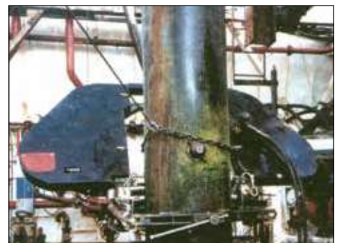
▼ Decommissioning job with band saw.
