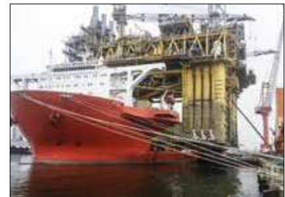
Synchronous superlift and launch
