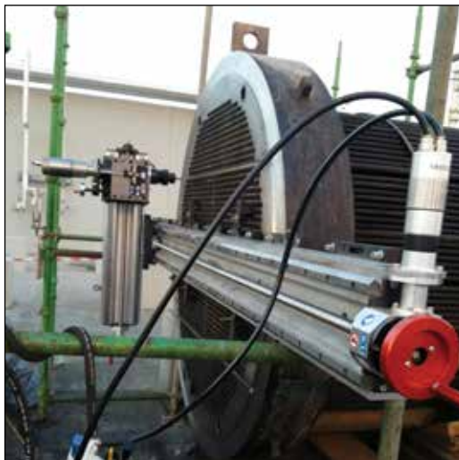
▼ MRY Milling machine on a heat exchanger.
