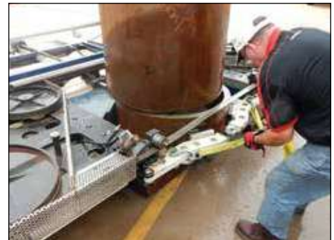
▲ Pipe cutting with BS portable band saw.
