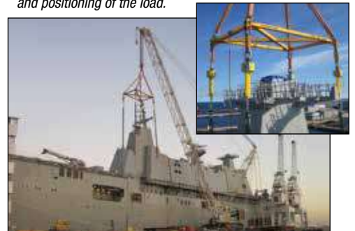
▼ A SyncHoist system used to align steel blocks of the ship's control tower sections allowing gradual lifting and positioning of the load.
