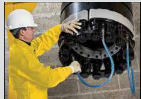
▲ Multi-Stud Tensioning application.
