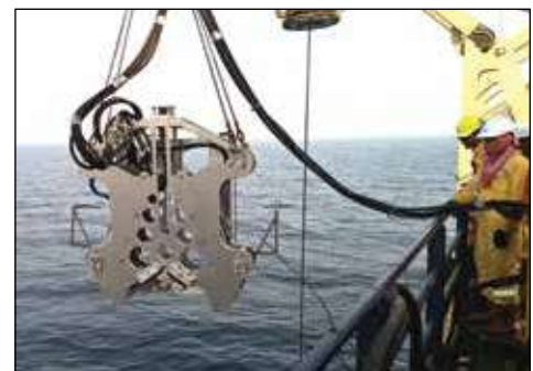
▲ MDWS Diamond Wire Saw lowered into sea.
