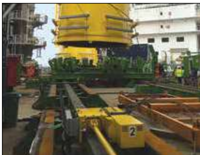
▼ The trolley system speeds up offshore wind transition piece load out: the transition pieces are positioned in the clamping frames and moved along the track.
