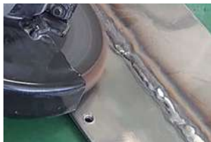
Removing blue weld discoloration
