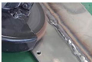
Removing blue weld discoloration
